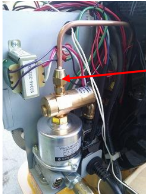
Picture 4 Inspection fuel pump
