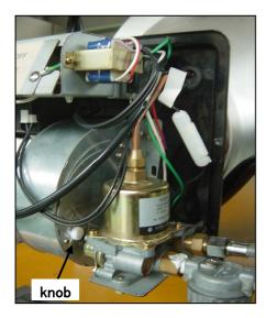
1. Unfasten a knob and expand combustion air inlet opening.
